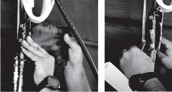
2. Now, place the supplied insulation material over the connectors and exposed refrigerant piping
