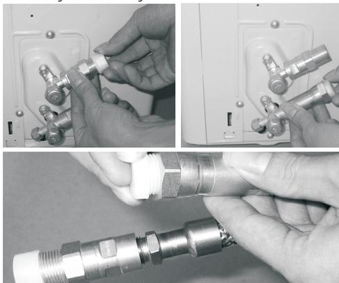
**NOTE: Ensure the adapters attached to the outdoor valves have been tightened properly before attempting to connect the line set.**
