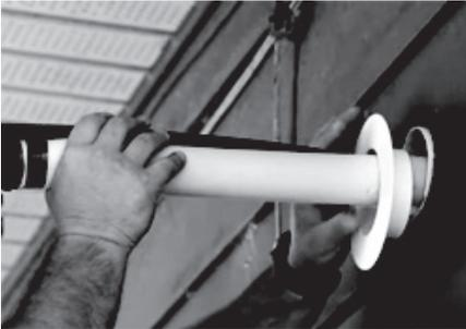
2. Place your hand on the underside of the piping coming through the exterior wall hole (from indoor unit), close to the wall. With your other hand, using even pressure, carefully bend the piping downward toward the wall, being mindful not to damage or dent the piping in the process.
