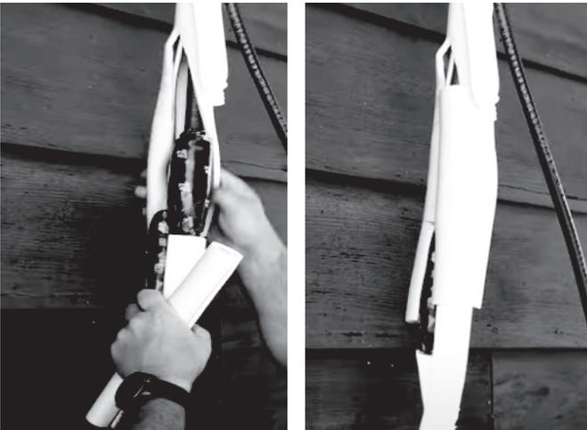
3. Now, starting where the line set is not covered with the factory plastic (close to the indoor air handler connection), you will wrap the line set upward to the wall hole, using the supplied Non-adhesive U.V. tape. This will cover the insulated line set connections, cables, and drain hose. The drain pipe will need to be at the bottom of the bundle (**Refer to Fig. 7.2**).
